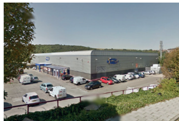
Large industrial unit to the west off Moulsecroomb Way.
