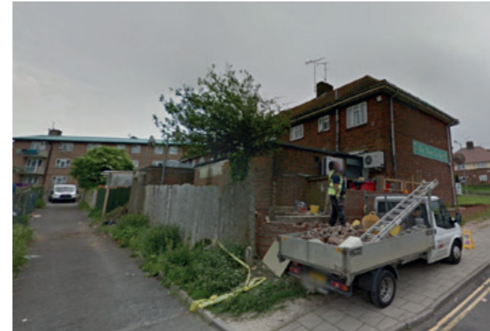
Rear of retail units with residential apartments above along Moulsecroomb Way
