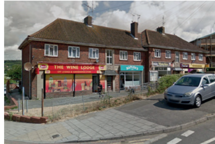
Retail units with residential apartments above along Moulsecroomb Way
